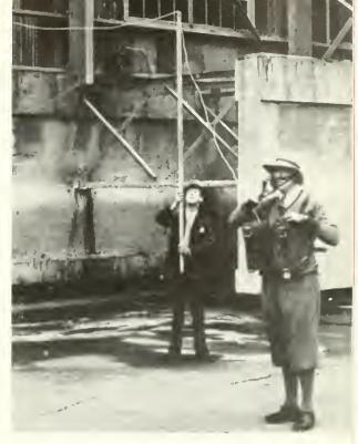
THIS EARLY VERSION OF THE PORT-ABLE TRANSMITTER WAS LARGE AND CUMBERSOME AND REQUIRED A LENGTH OF WIRE FOR ITS ANTENNA.
