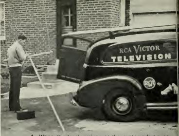
4. When the truck arrives at the customer's house, the RCA dipole receiving antenna is assembled an the ground before being erected on the roof.
