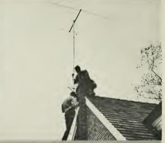
Using special rigging and supports, the antenna is clamped securely to the most suitable spot on the roaf.
