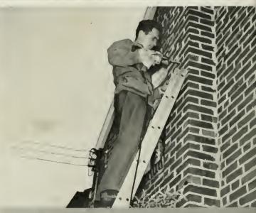
Holes are drilled in the slde of the house to support hooks for the RCA "Bright-picture" tape which conveys signals to the receiver.
